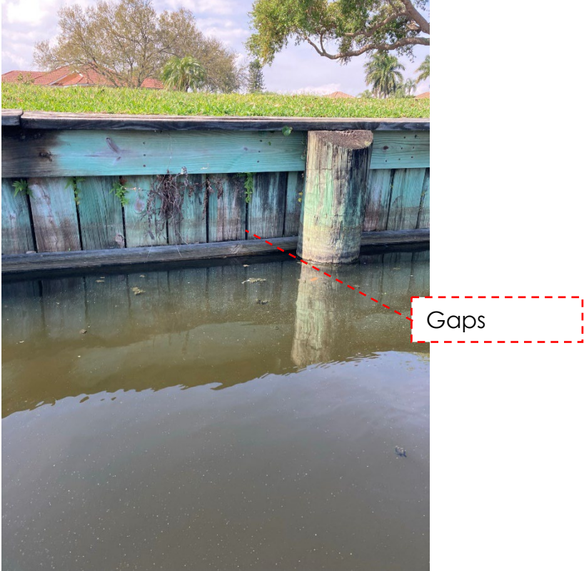
Photo 6: View of Gaps Between Vertical Boards
