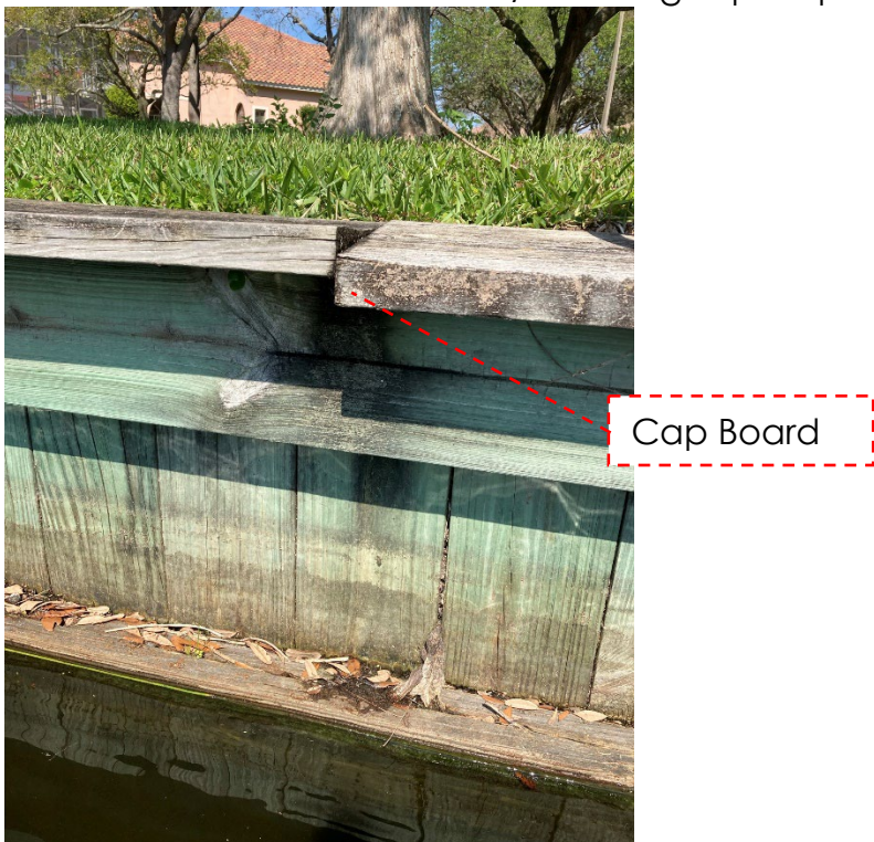
Photo 2: View of Deteriorated/Cracking Top Cap
