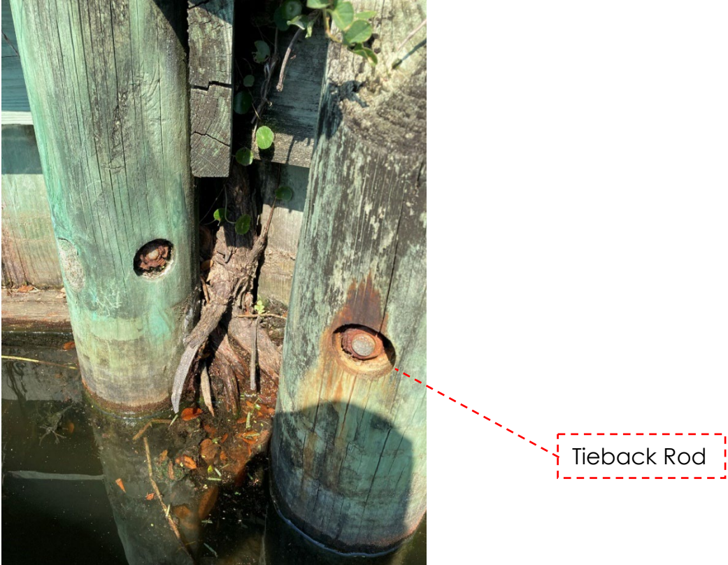
Photo 4: View of Corroded Tieback Rods
