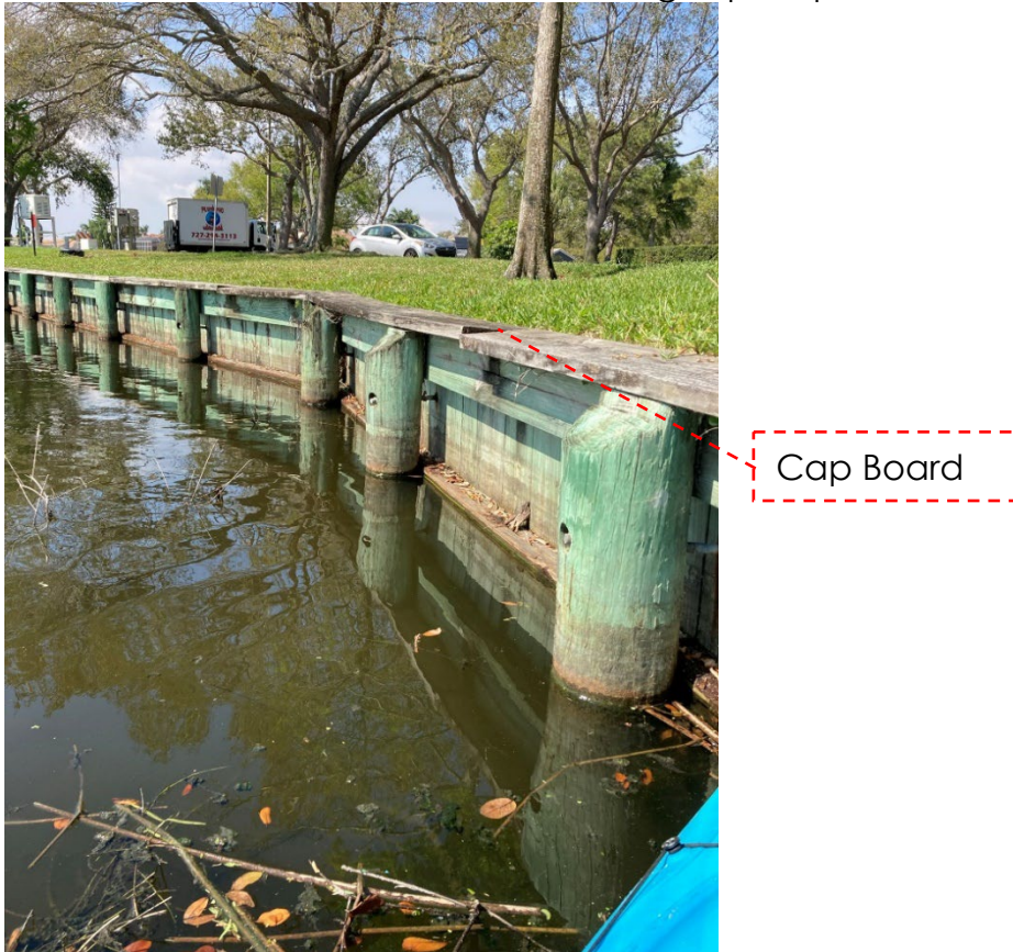
Photo 2: View of Deteriorated/Cracking Top Cap
